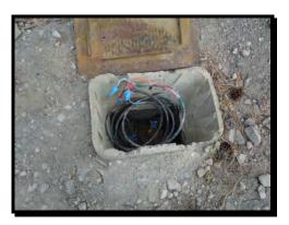
• Replaced a damaged G-5 Box on the side of Village Hall.
