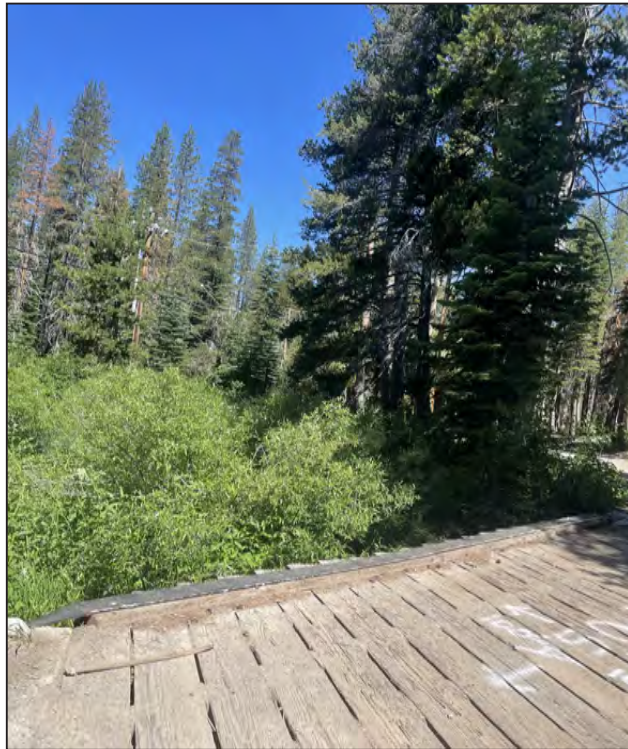
Photo 3: Crossing of perennial drainage (South Yuba River) and riparian area, facing northwest.
